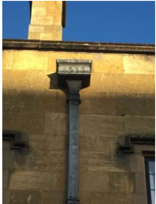
Figure F2: Cast Iron pipes with hopper detail. 1935 construction date illustrated on hopper. Source: Site Visit, 30 th November 2018.
