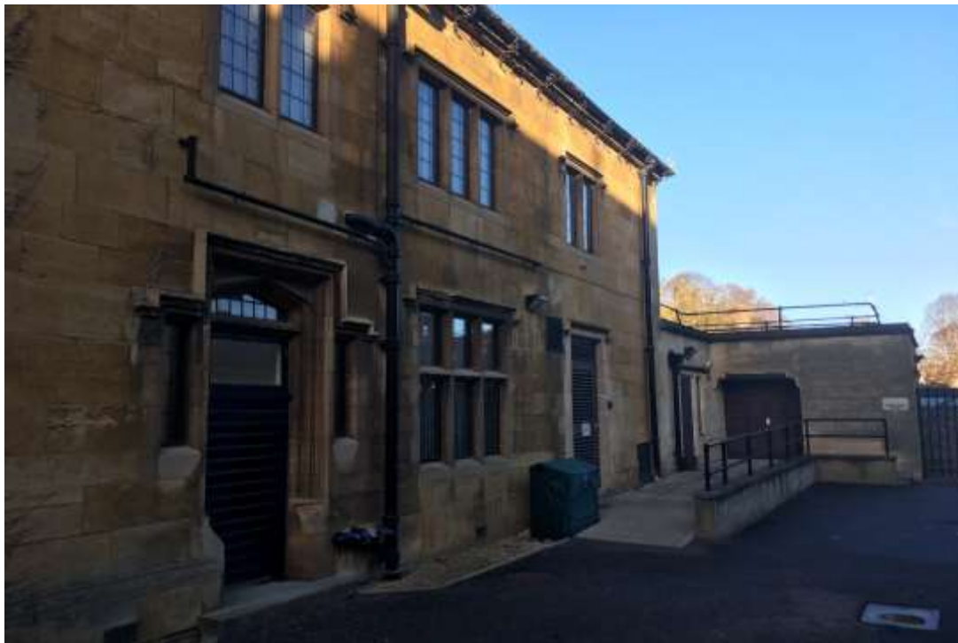
Figure F3: East Elevation of Banbury Magistrates Court. The rear extension is not original. Windows/doors have undergone numerous alterations, although detailing/changes have been sympathetic to the original design. Source: Site Visit, 30 th November 2018.
