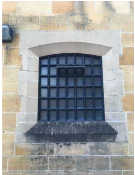
Figure F5: Cell window, rear/west elevation. Exterior retained but false windows infilled behind. Source: Site Visit, 30 th November 2018.
