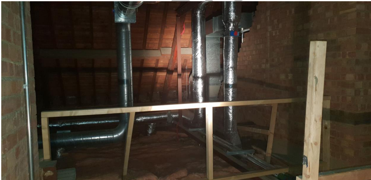
Image 6 – Internal view from central area of roof void demonstrating a timber cladding below the tiled coverings along with an insulated covering to the floor area
