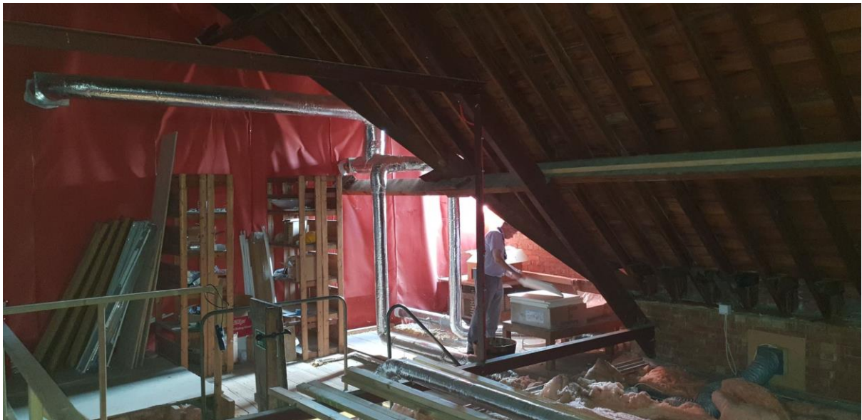
Image 7 – Further views from within the roof void demonstrating the air-conditioning pipework's running within the void areas along with plastic sheetings
