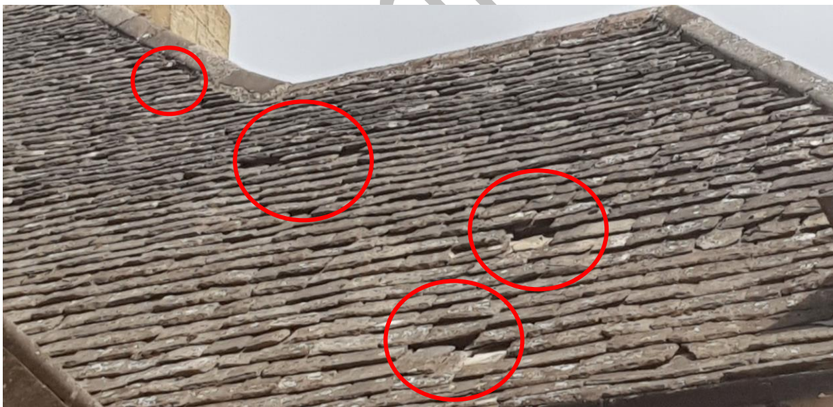
Image 2 – Areas of deterioration to the roof coverings (South facing) have been identified to include missing tiles and gaps to the ridge tiles which offer roosting value to bats
