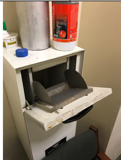
Photo 10: Example of Asbestos Insulating Board panel within incinerette
