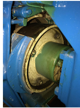
Photo 8: Brake pads to lift motor (Third Floor, Lift 6 Motor room)
