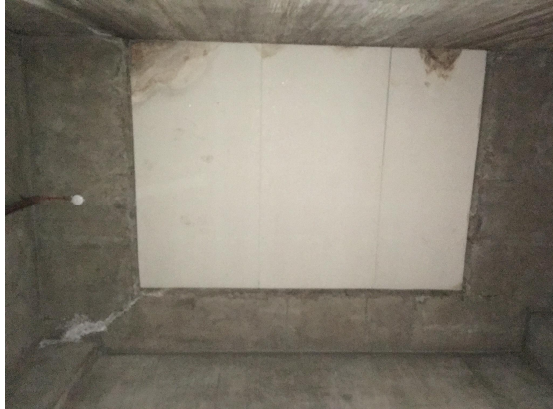
Photo 29: Basement Boiler House ceiling, non-asbestos insulating board (with possible sprayed coating behind)
