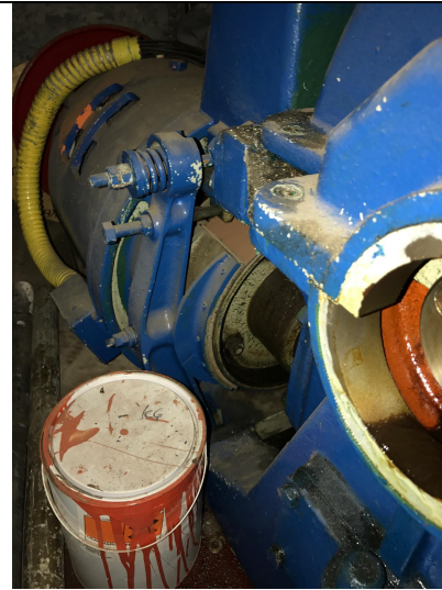
Photo 26: Brake shoes to redundant lift motor
