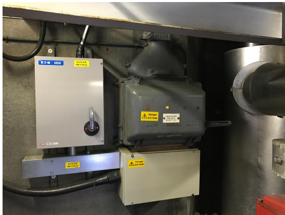
Photo 9: Example of Woven textile flashguards within electrical box
