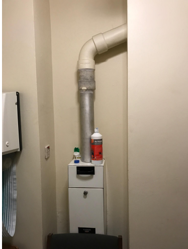
Photo 11: Example of cement flue pipe to incinerator
