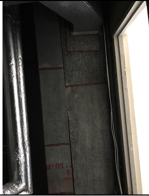
Photo 7: Example of red/brown mastic to air handling unit
