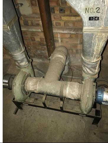
Photo 24: Gaskets to hot pipework
