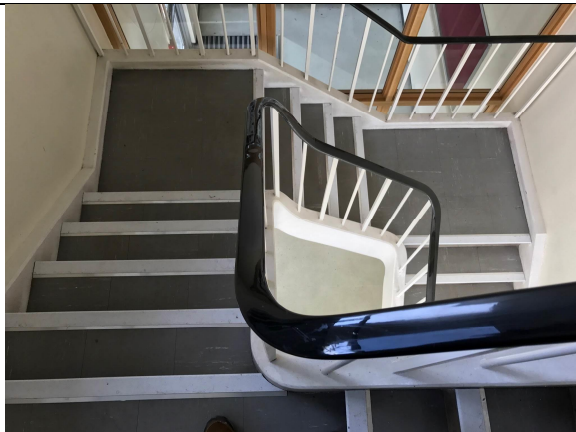
Photo 15: Stair Nosing and Vinyl floor tiles (First Floor, Staff stairs)
